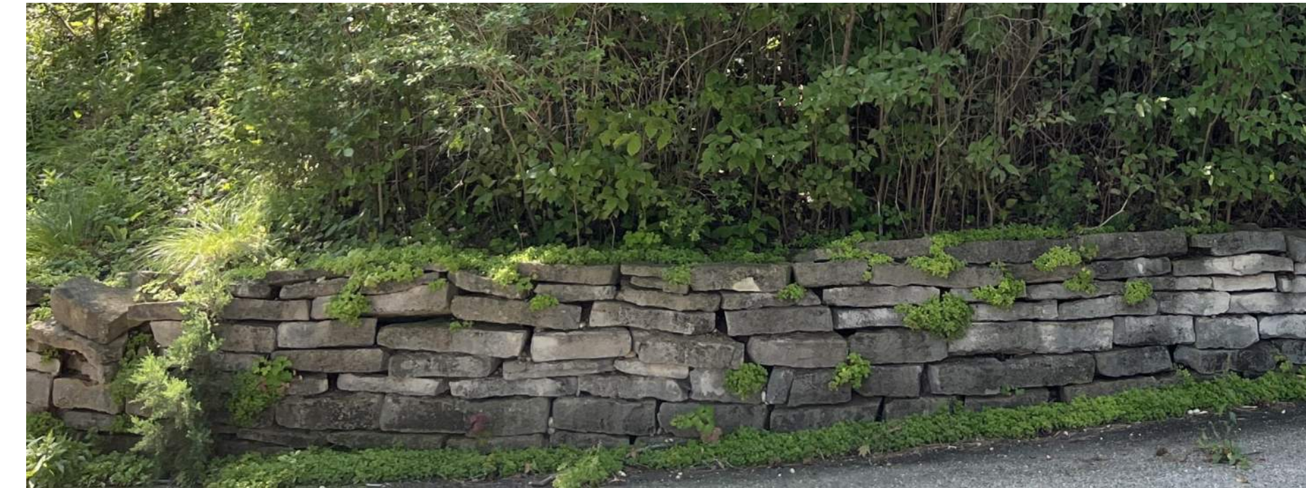
EXISTING DRY STACK WALL
