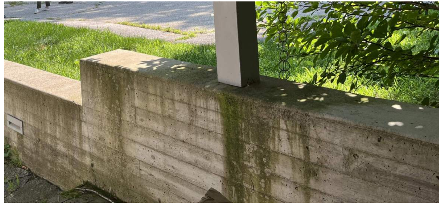
EXISTING BOARD FORMED CONCRETE WALL
