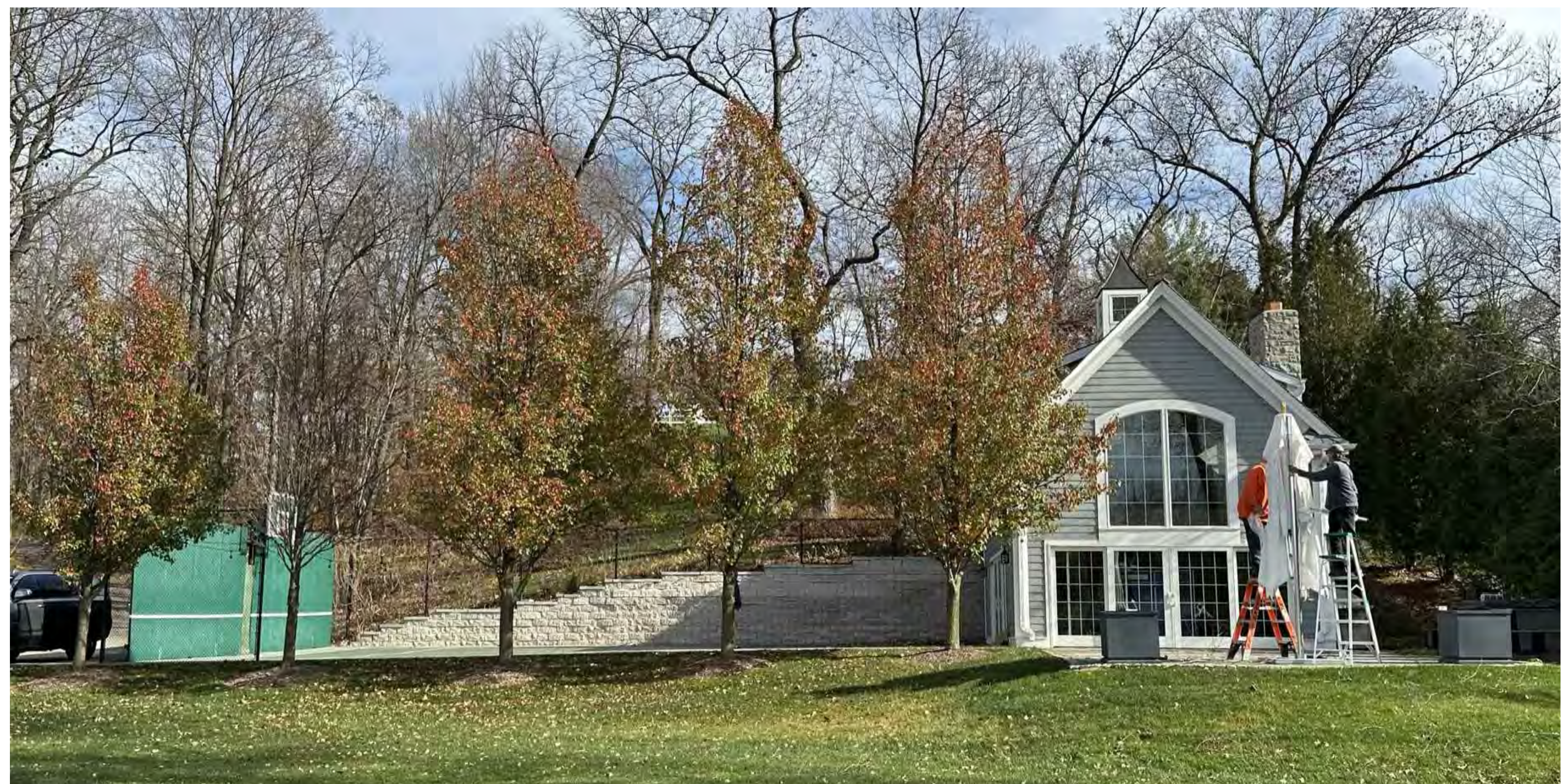
EXISTING CONDITION PHOTO LOOKING EAST - 11.09.22
