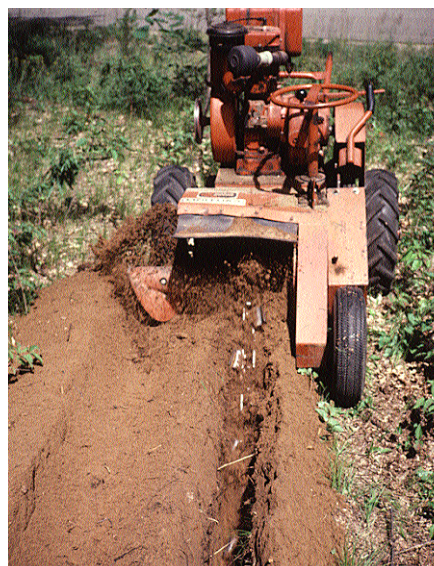
Example 3b. Oak wilt trenching.
