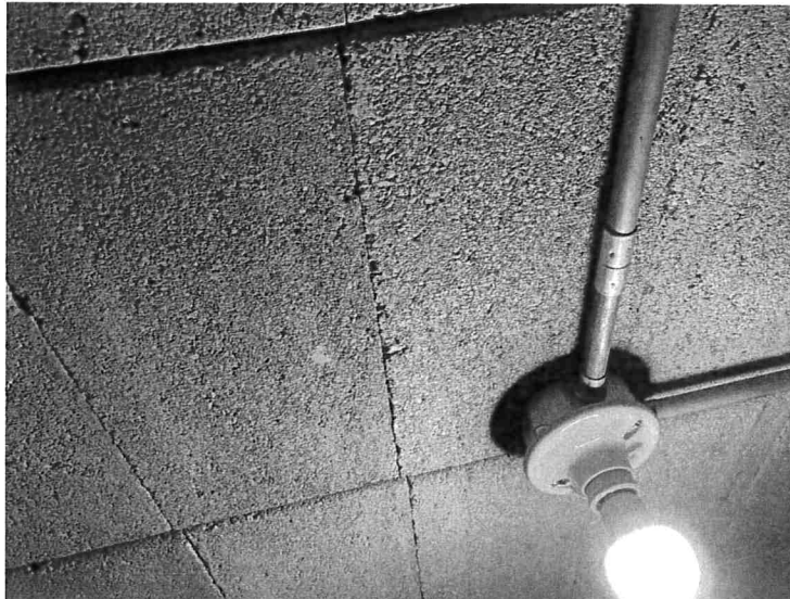
Existing Dox Block Ceiling in Lower Level
