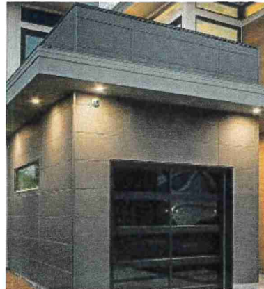
Nichiha "Toughblock Steel" Siding 72" x 18" panels
