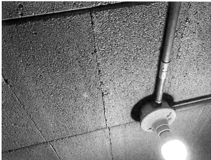
Existing Dox Block Ceiling in Lower Level
