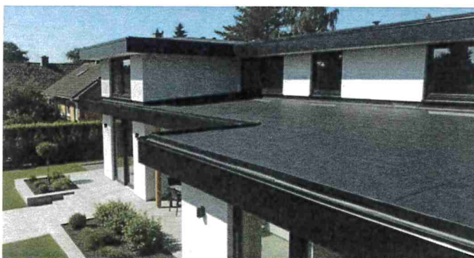
EPDM Rubber Roofing; Aluminum Metal Fascia Materials (20" tall), black
