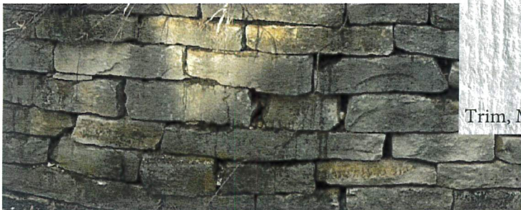
Retaining Wall -Match Ex.
