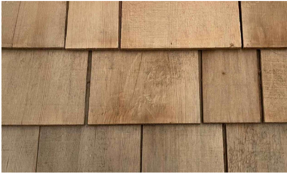
CEDAR ROOF SHINGLES PRECISION CUT CEDAR ROOF SHINGLES WITH 5" EXPOSURE
