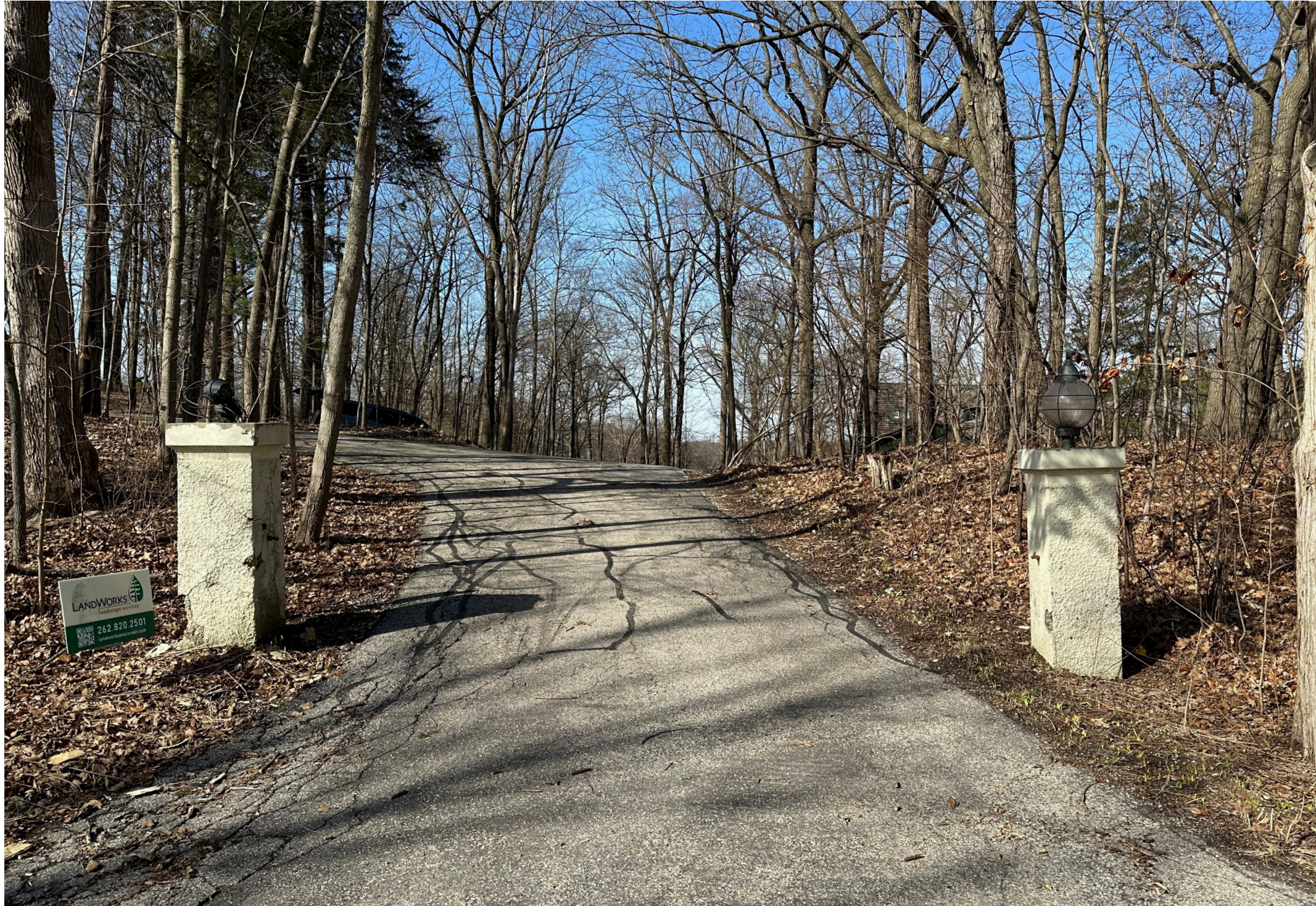
EXISTING ENTRY PILLAR DIMENSIONS: 1'-8 1/2" x 1'-8 1/2" x 7'-3" (top of light fixture) 4'-9" (top of masonry cap)
