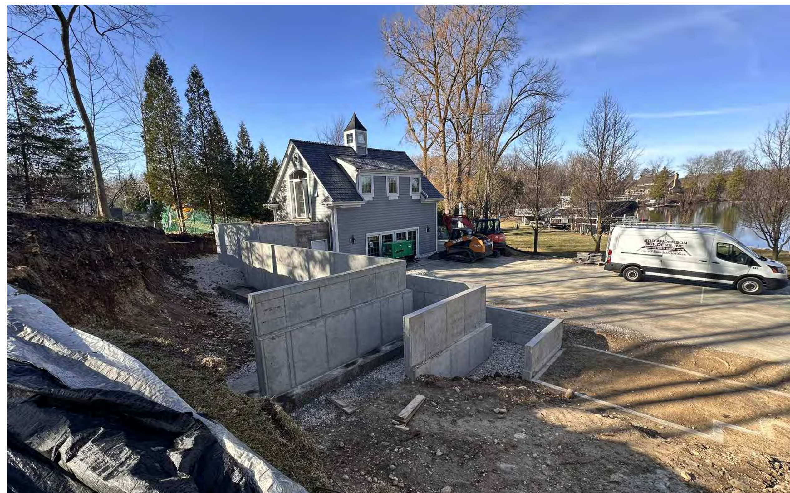
CONSTRUCTION PHOTO LOOKING SOUTHEAST - 03.13.24
