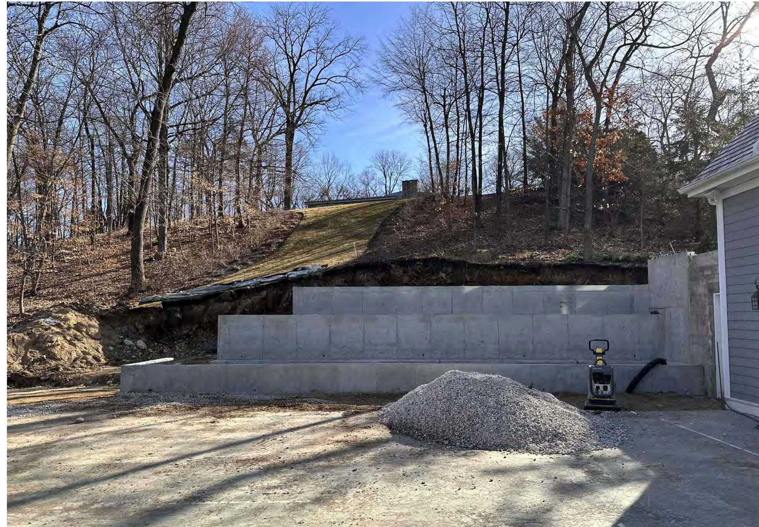
CONSTRUCTION PHOTO LOOKING SOUTHEAST - 03.13.24
