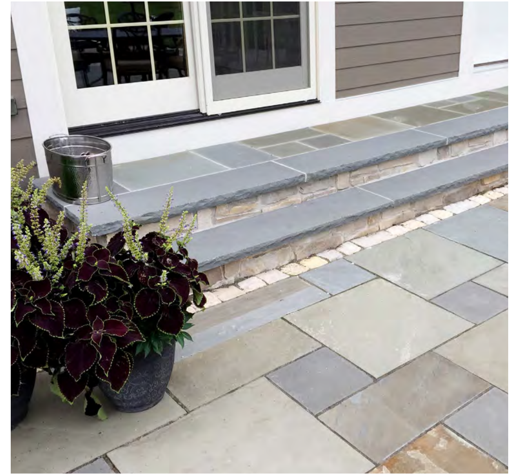
Pattern Bluestone Stone Patio and Steps
