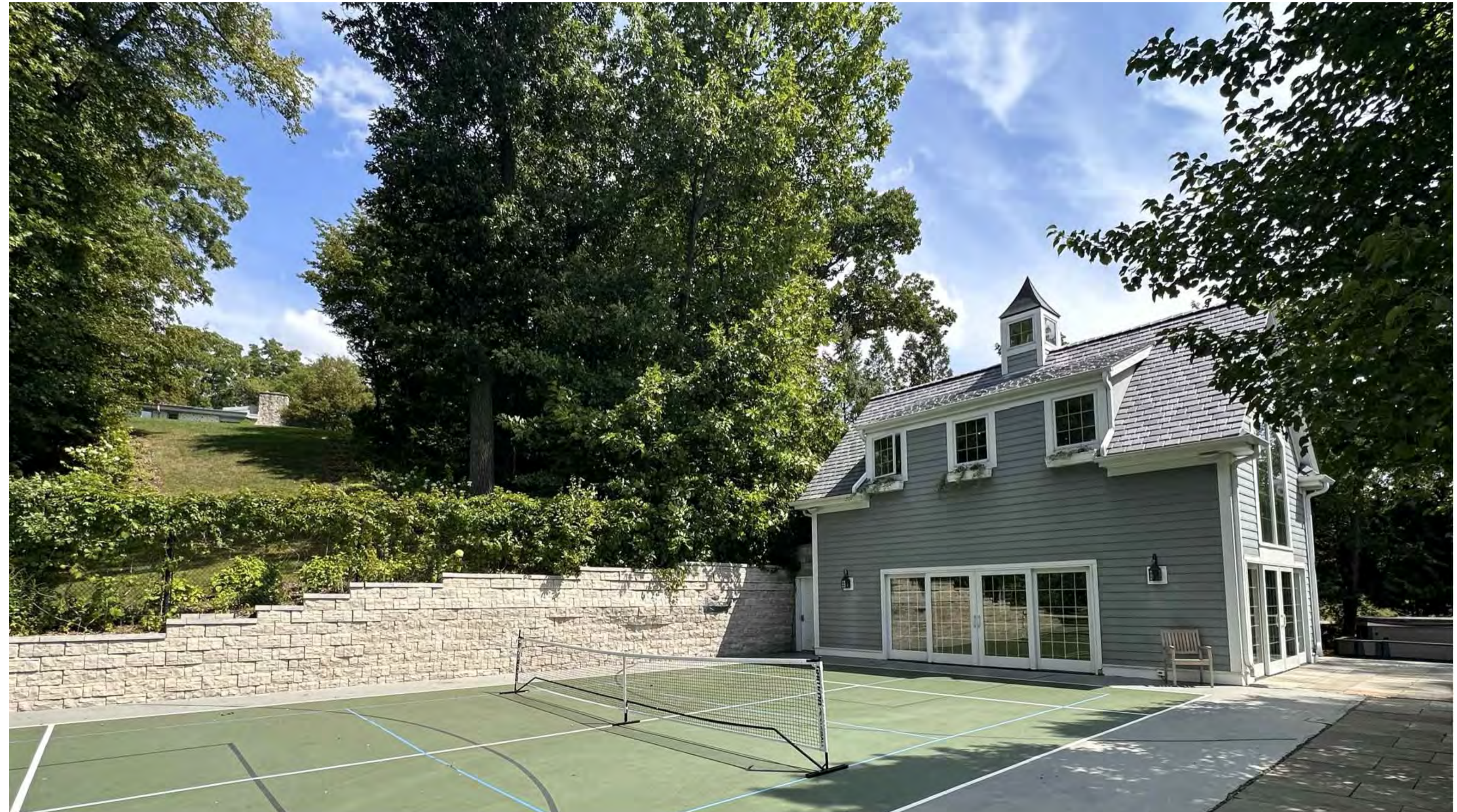
EXISTING CONDITION PHOTO LOOKING SOUTHEAST - 08.07.23
